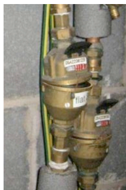
Figure 4: Lack of insulation will allow internal water meters to freeze and split causing a loss of water supply
