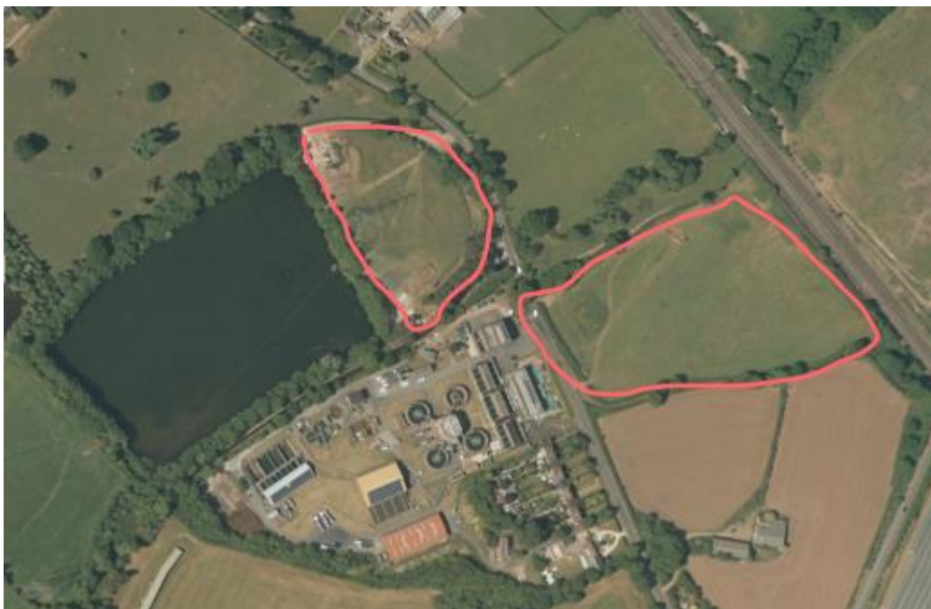
2 locations (both SSC owned) – totalling 2.5 MWp ground mounted PV (No export)
