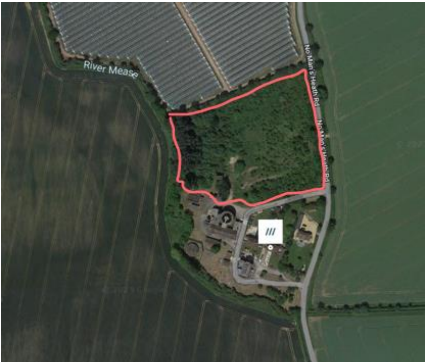
Field alongside pumping station - 0.3 MWp ground mounted PV (No export)
